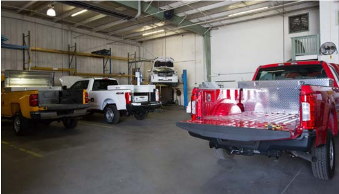
This CNG vehicle conversion facility is outfitted with a fuel-leak mitigation system. The system includes the in-wall exhaust fan shown in the upper right. Photo by Amy Glickson, NREL 45006
